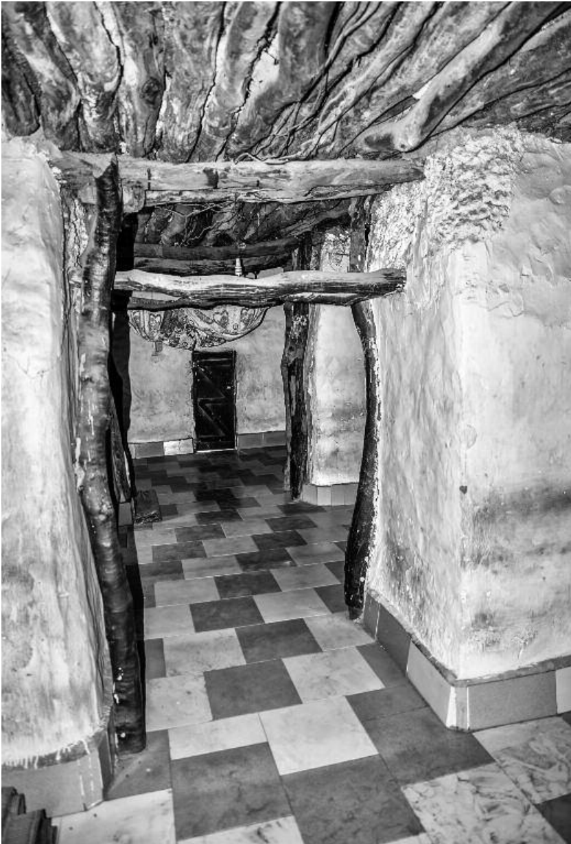
Fig. 45 Banda Nkwanta, detail of the wooden beams linking the pillars together and with the lateral walls inside the prayer hall (photo Denis Genequand).
