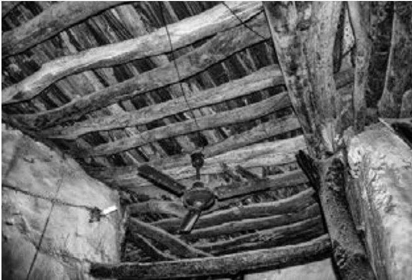
Fig. 38 Bole, detail of the roof of the prayer hall: wooden beams, joists and roof battens with alternating orientation (photo Denis Genequand).
