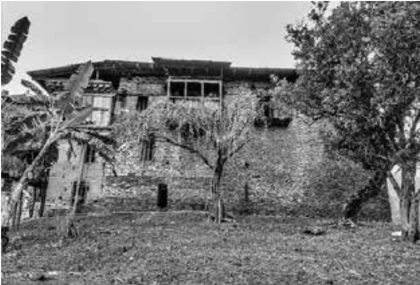
Fig.2 Northern wall of the Khoche manor in Bjoka
